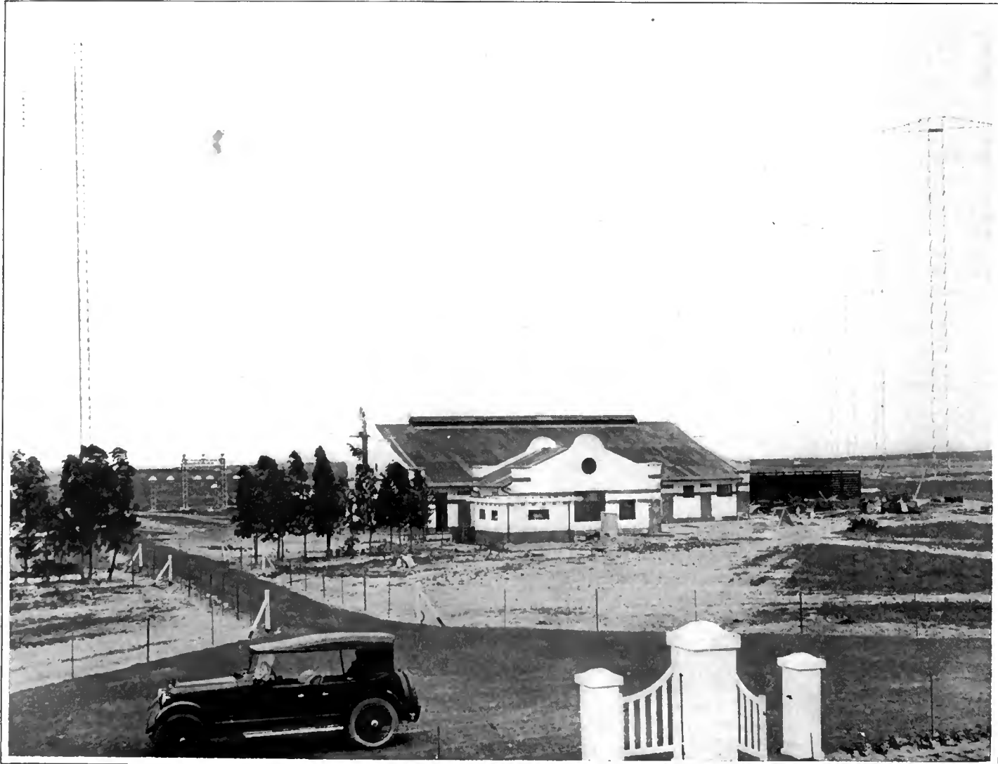
THE MARCONI SOUTH AFRICAN BEAM STATION
